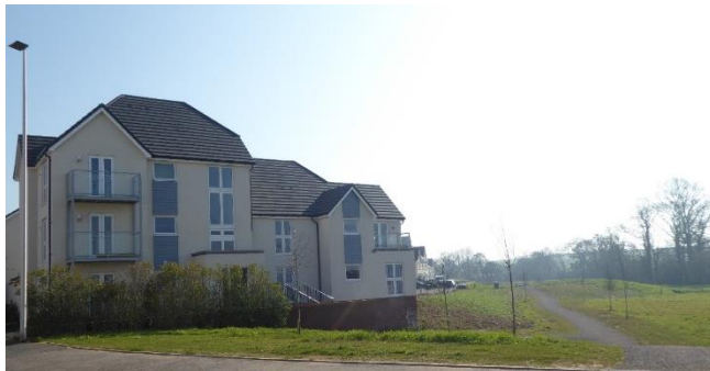
Affordable housing overlooking the country park in Cranbrook
