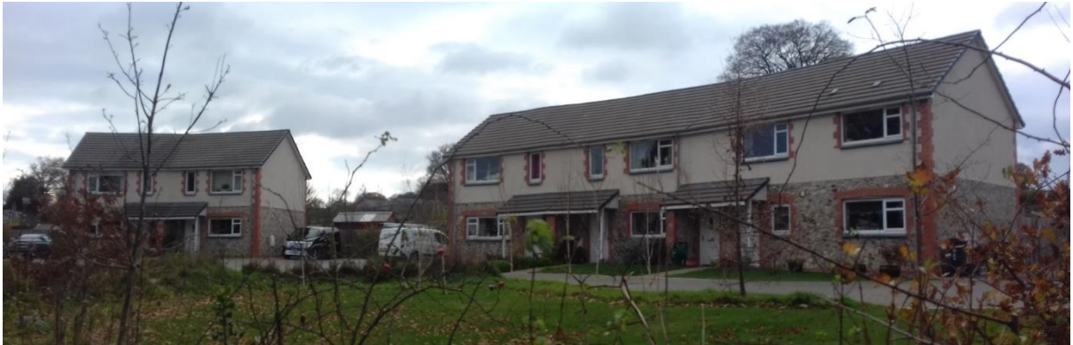
Six affordable homes on a rural exception site in Dalwood, delivered by Corry Valley Community Land Trust
