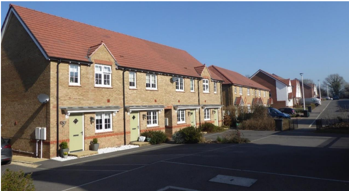
A terrace of four affordable homes, part of a larger housing development in Ottery St Mary
