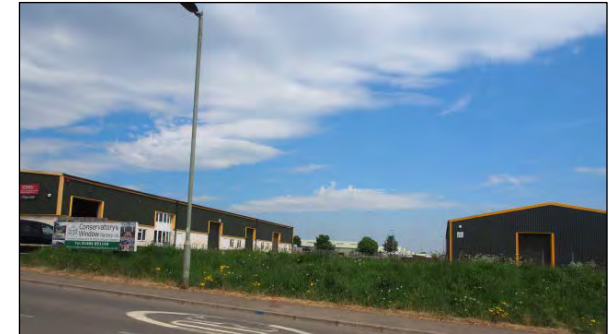
New industrial buildings adjacent to Dunkeswell Airfield
