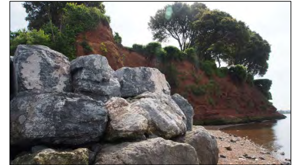
Rock armour protecting eroding headland, Exe Estuary
