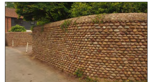
Modern wall using traditional materials and techniques, Colaton Raleigh, near Bicton
