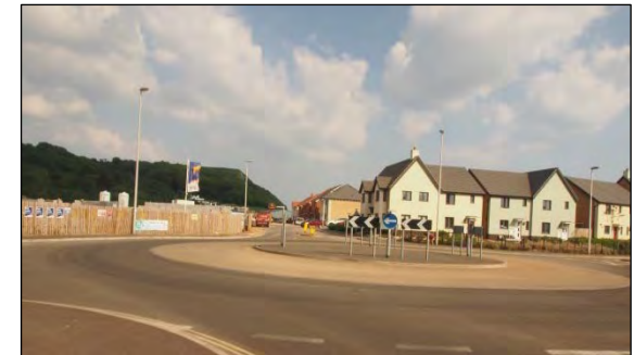
New development on former coastal plain at Seaton (now classified as 'urban')
