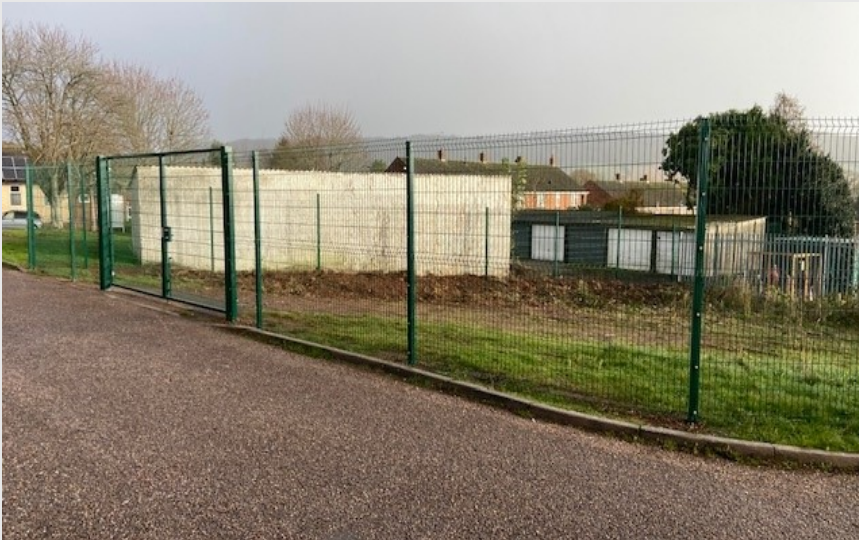
New Compound at Manstone Workshops
