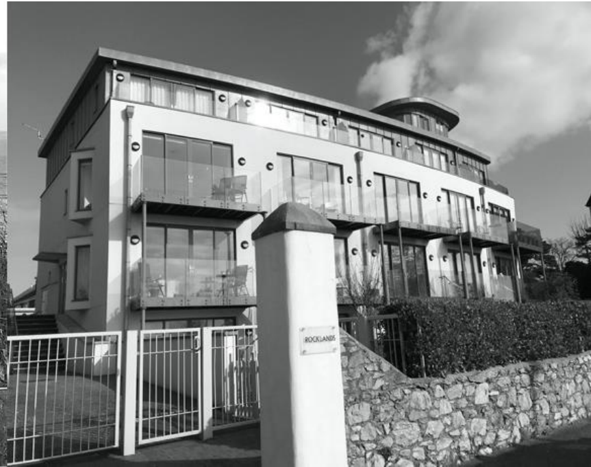
Rocklands – windows and balconies
