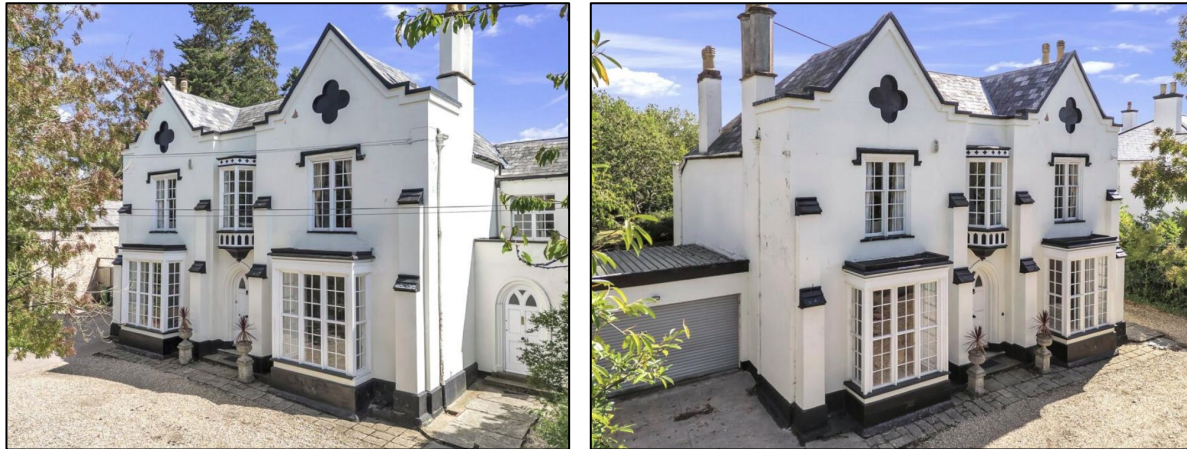
Burwood Principal Gothic Elevation following roof repairs
