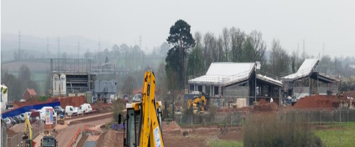
Construction at Cranbrook
