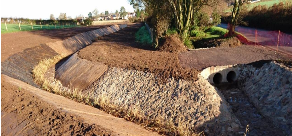
Flood alleviation works at Feniton
