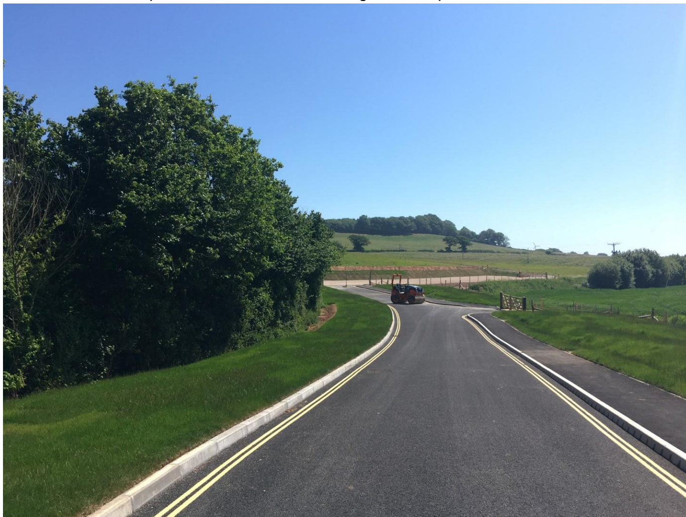
Photo 3. Works completed on access road, drainage and car park.
