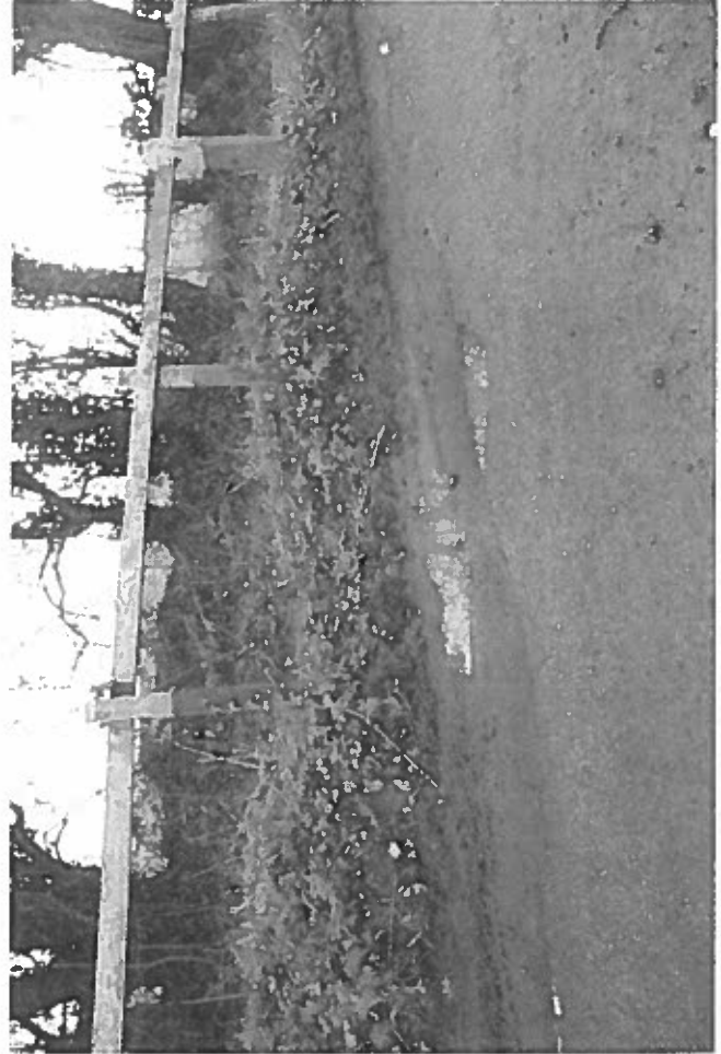
Channel needs to be dug to allow road to drain
